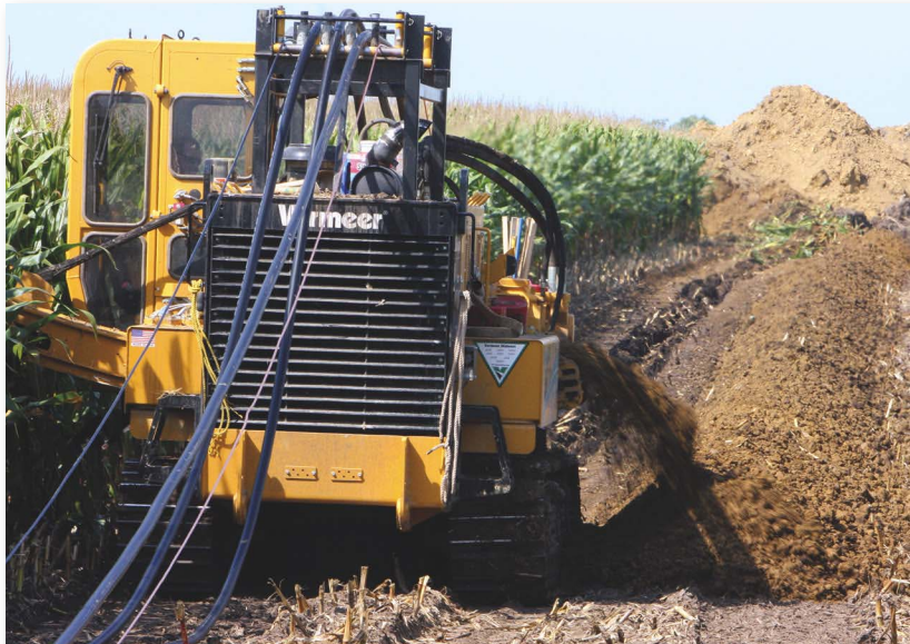
With the Vermeer CL80 cable layer attachment, a series of rollers takes the multiple cables required for wind-energy transmission, guides them over the machine, and feeds them into a cable box where they are sorted in the appropriate configuration.
